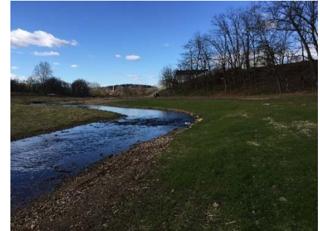
After construction, the streambanks are gradual. After this photo was taken, more than 2,000 native trees and shrubs were planted.
