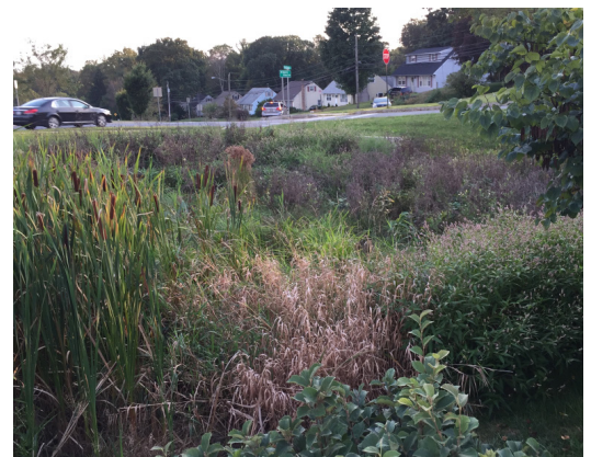
Without proper maintenance, weeds will take over stormwater management basins as shown above.
