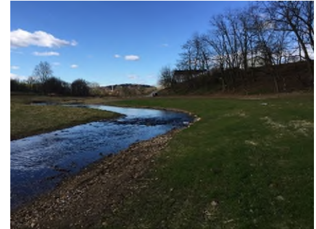
After construction, the streambanks are gradual. After this photo was taken, more than 2,000 native trees and shrubs were planted.
