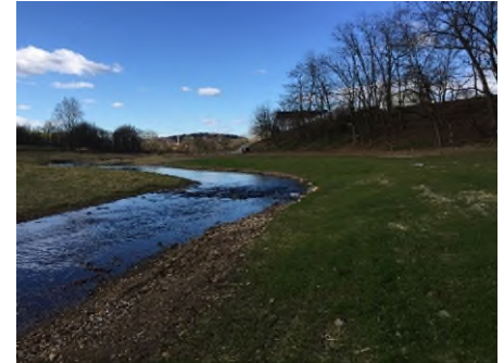
After construction, the streambanks are gradual. After this photo was taken, more than 2,000 native trees and shrubs were planted.
